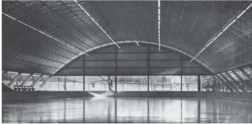
Figure 1.8 Cold-formed steel members used in a 100 \times 220 \times 30 -ft ( 30.5 \times 67.1 \times 9.2 -m) tridetic arch. Courtesy of Butler Manufacturing Company.
