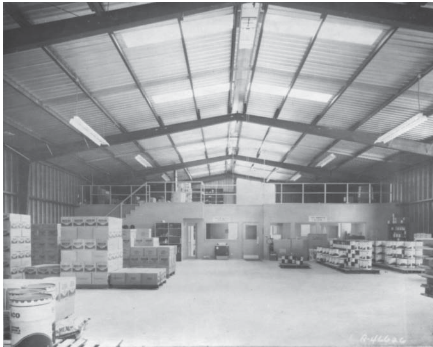
Figure 1.21 Standardized building made of fabricated rigid frame with cold-formed sections for girts, purlins, roofs, and walls. Courtesy of Armco Steel Corporation.
