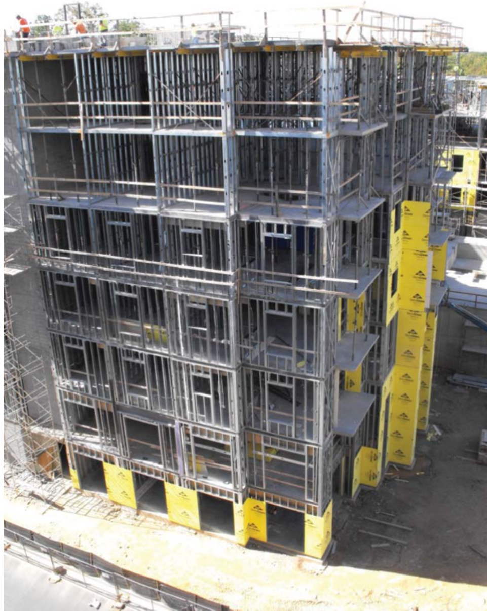
Figure 1.3 Building composed entirely of cold-formed steel sections. Courtesy of Don Allen.
