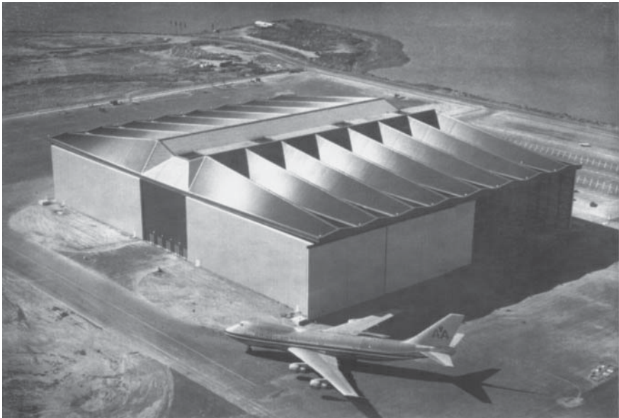
Figure 1.15 Super bayhangar for American Airlines Boeing 747s in Los Angeles. 1.82 Courtesy of Lev Zetlin Associates, Inc.
